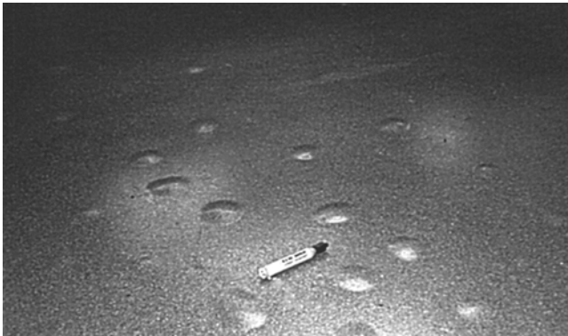
Fig. 1.2—Blisters due to moisture in concrete. (Courtesy of Peter Craig.)
