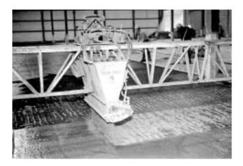
Fig. 8.3—Mechanical spreader.
