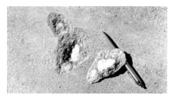
Fig. 11.7—A popout is a small fragment of concrete broken away from the surface of a slab due to internal pressure, leaving a shallow, typically conical, depression (PCA 0113).
