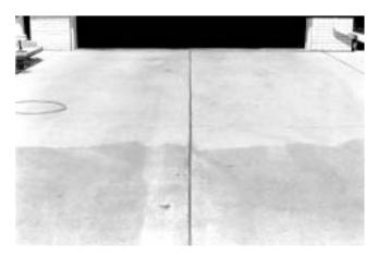
Fig. 5.1—Concrete slab discoloration due to the use of calcium chloride mixture. Concrete in upper part of the photo did not contain the admixture.
