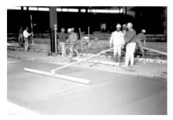
Fig. 8.6—"Modified highway" straightedge.
