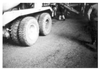
Fig. 4.1—Proof-rolling by loaded ready mix truck.
