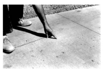
Fig. 11.3—Crazing is a network of very fine superficial surface cracks (PCA 4099).
