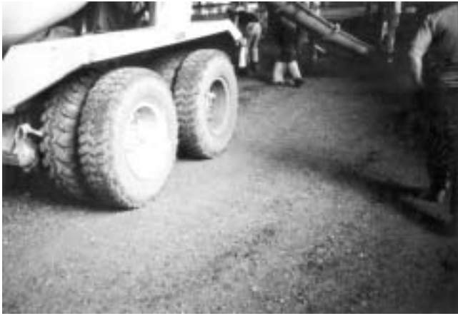
Fig. 4.1—Proof-rolling by loaded ready mix truck.
