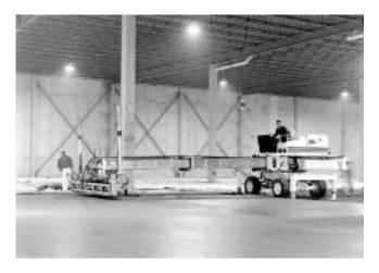
Fig. 8.4—Laser-controlled screed.
