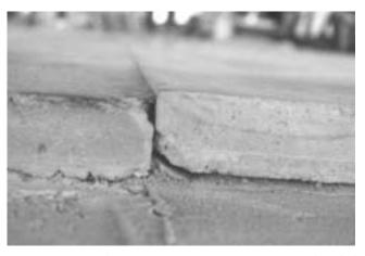
Fig. 11.12—Curling at joint in a 2 in. (50 mm) unbonded topping (courtesy of Eldon Tipping).
