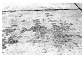
Fig. 11.5—Scaling is the loss of surface mortar, usually exposing the coarse aggregate (PCA A5273).
