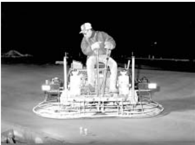
Fig. 8.5—Double-riding trowel with clip-on pans.
