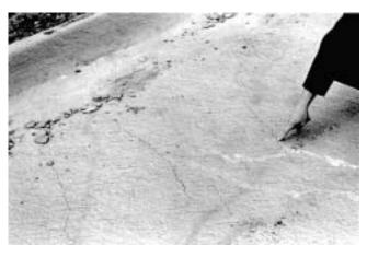
Fig. 11.2—Plastic-shrinkage cracks are caused by rapid loss of mixing water from the surface while the concrete is still plastic (PCA 1311).
