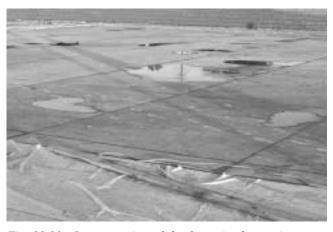
Fig. 11.11—Low spots in a slab after rain shower (courtesy of Eldon Tipping).
