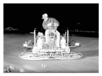
Fig. 8.5—Double-riding trowel with clip-on pans.
