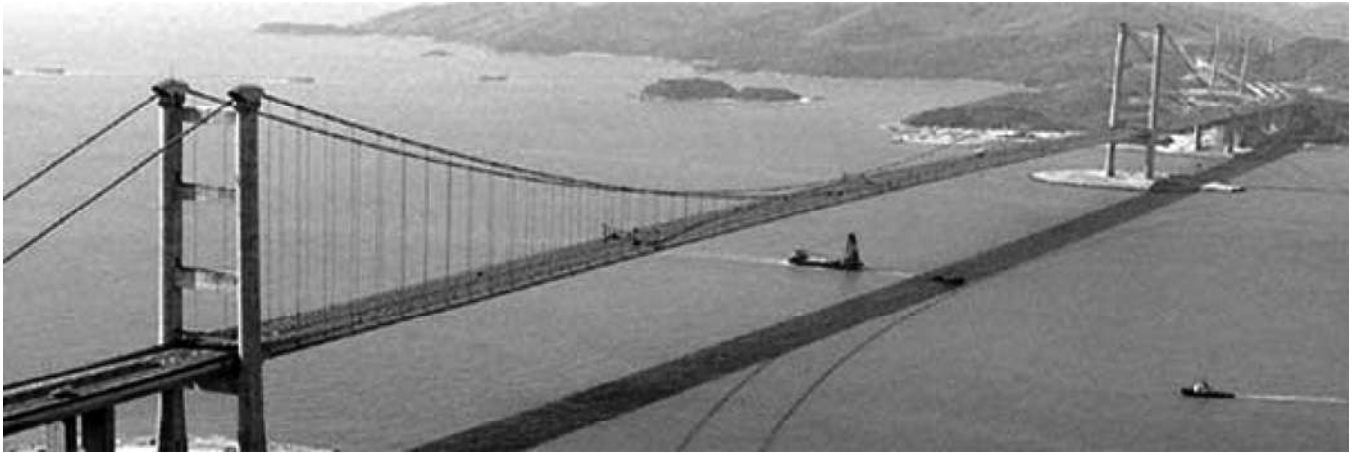
Fig. 6.1—Tsing Ma Bridge, Hong Kong.
