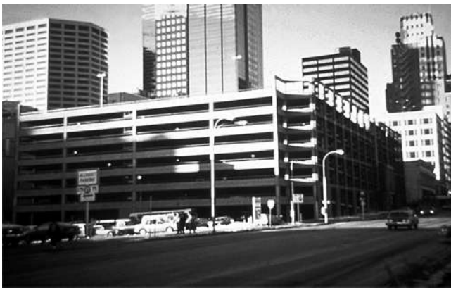
Fig. 6.8— Town Pavillion Parking Garage, Kansas City, Mo.
