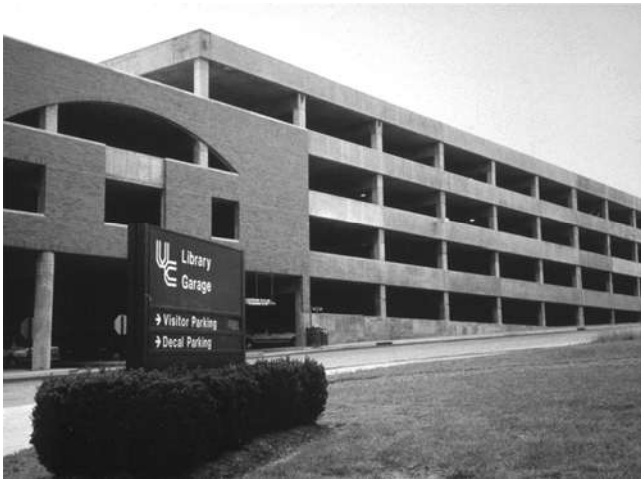
Fig. 6.7— Administration Parking Garage at University of Cincinnati, Ohio.
