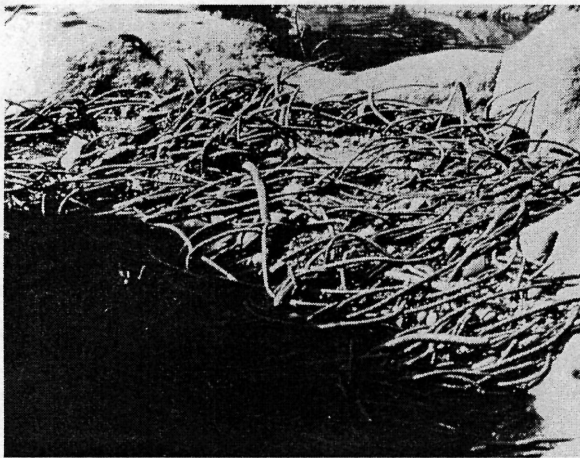
Fig. 3.3-Typical debris resulting from abrasion erosion of concrete
