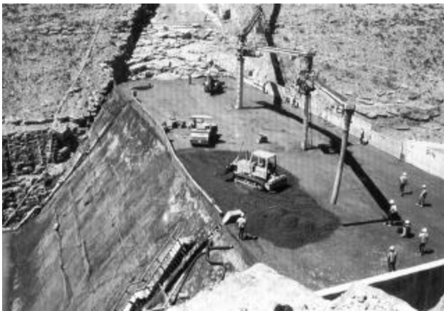
Fig. 5.2—All-conveyor system supported on posts in dam.
