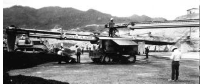
Fig. 5.3—All-conveyor system utilizing crawler placer.
