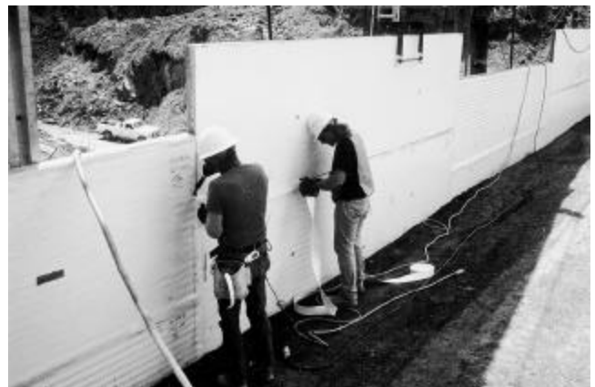
Fig. 4.8—Installation of precast facing panel with attached membrane.
