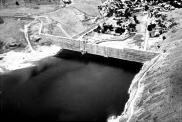
Fig. 1.1—Willow Creek Dam.
