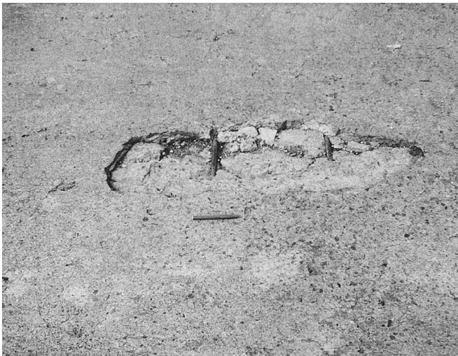
Fig. A.2.9—Delaminations
