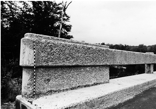
Fig. A.2.20.3a—Scaling (severe)
