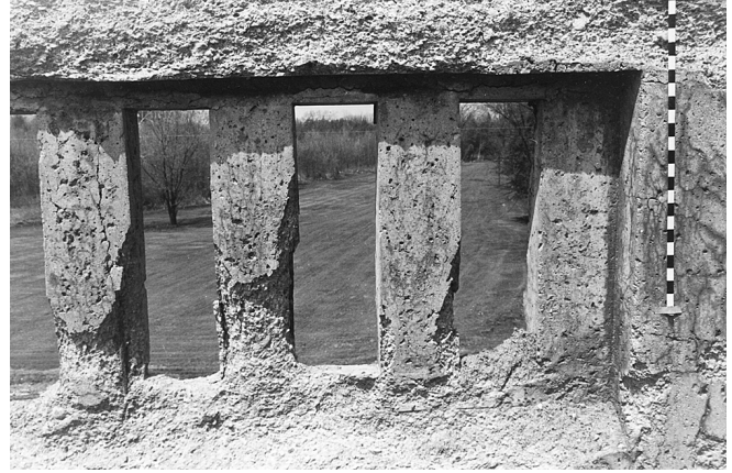
Fig. A.2.20.4a—Scaling (very severe)
