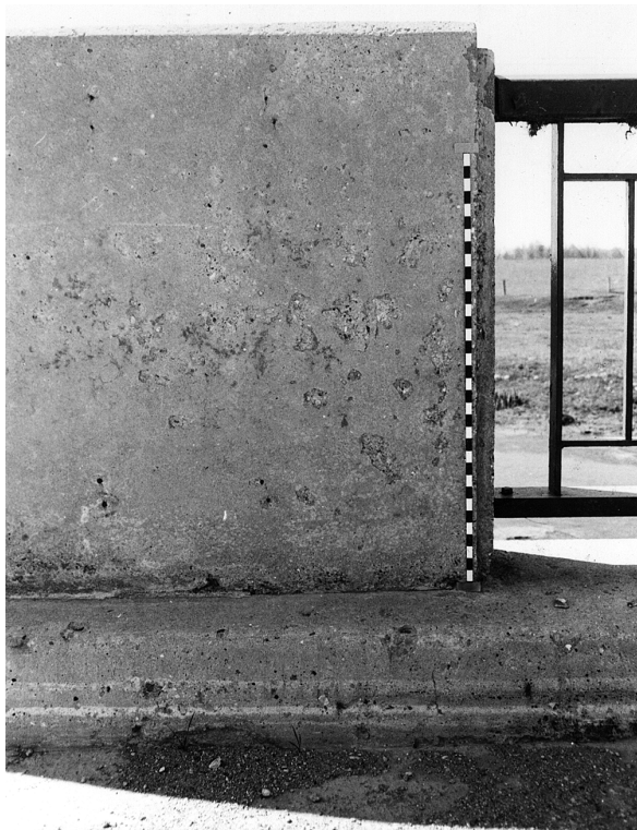
Fig. A.2.20.1a—Scaling (light)
